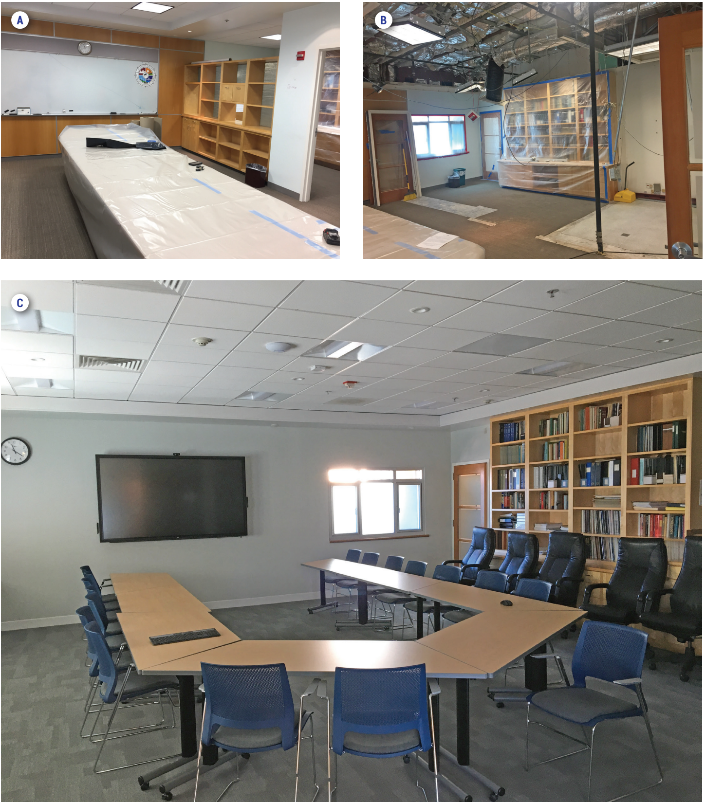
FIGURE 33: Boardroom remodel. (A) The boardroom prior to the remodel. (B) The boardroom after the removal of the partitioning cabinetry, dividing wall, and small corner supply room. (C) The remodeled boardroom is now a meeting space with modular furniture that can change configurations.
