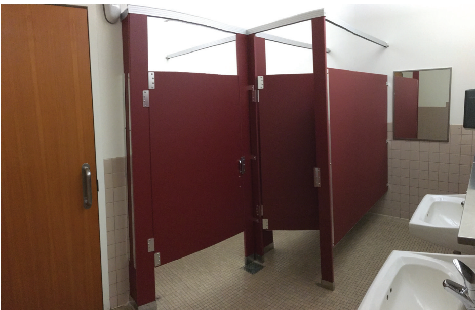
FIGURE 31: New bathroom partitions
