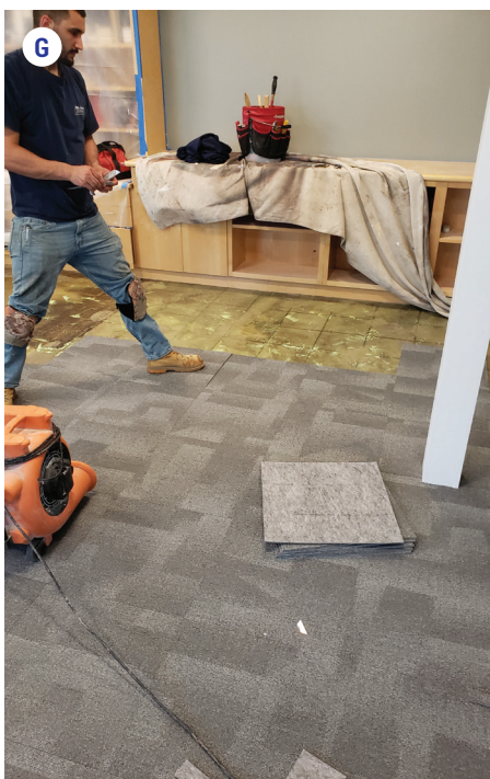
FIGURE 28: Updated flooring. (A) Reception area prior to flooring update with vinyl floors still intact. (B) Reception area during the flooring update. (C) Reception area after the flooring update with new polished concrete finish. (D) Laboratory during the vinyl removal process. (E) Laboratory during the new flooring process. (F) Laboratory with new chemical resistant flooring. (G) New carpet tile installation in meeting rooms and offices.
