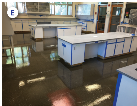
FIGURE 28: Updated flooring. (A) Reception area prior to flooring update with vinyl floors still intact. (B) Reception area during the flooring update. (C) Reception area after the flooring update with new polished concrete finish. (D) Laboratory during the vinyl removal process. (E) Laboratory during the new flooring process. (F) Laboratory with new chemical resistant flooring. (G) New carpet tile installation in meeting rooms and offices.
