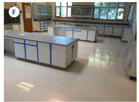
FIGURE 28: Updated flooring. (A) Reception area prior to flooring update with vinyl floors still intact. (B) Reception area during the flooring update. (C) Reception area after the flooring update with new polished concrete finish. (D) Laboratory during the vinyl removal process. (E) Laboratory during the new flooring process. (F) Laboratory with new chemical resistant flooring. (G) New carpet tile installation in meeting rooms and offices.
