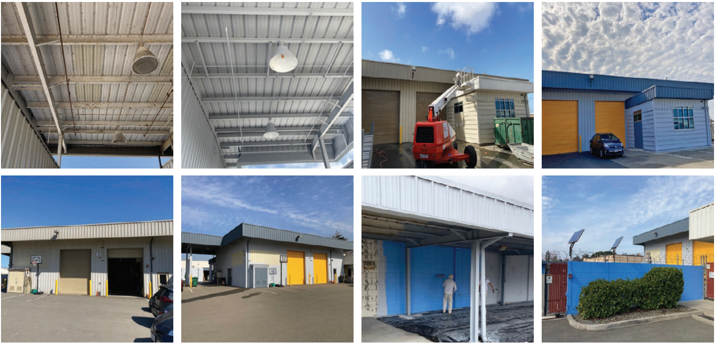
Figure 27. Before, after, and during the exterior paint project.
