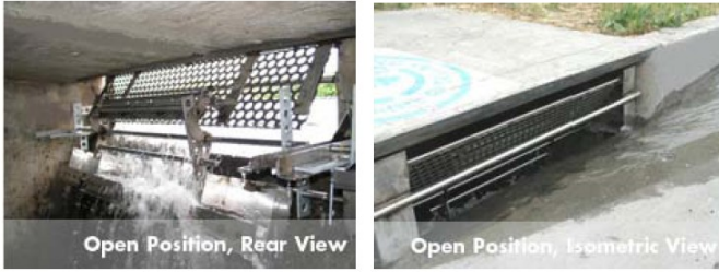
USW-2 Clean Screen III Automatic Retractable (inlet) Screen; ARS
