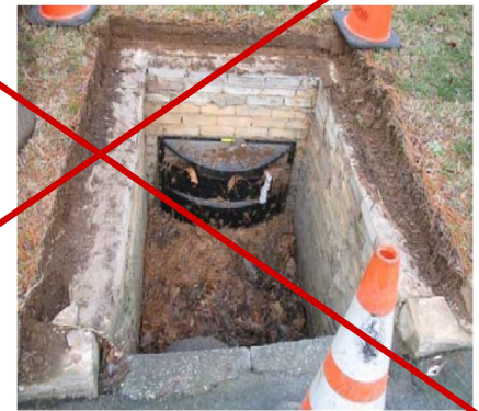
BC-4 Trash Guard Plastic (HDPE) catchbasin connector pipe screen. 3 standard sizes
