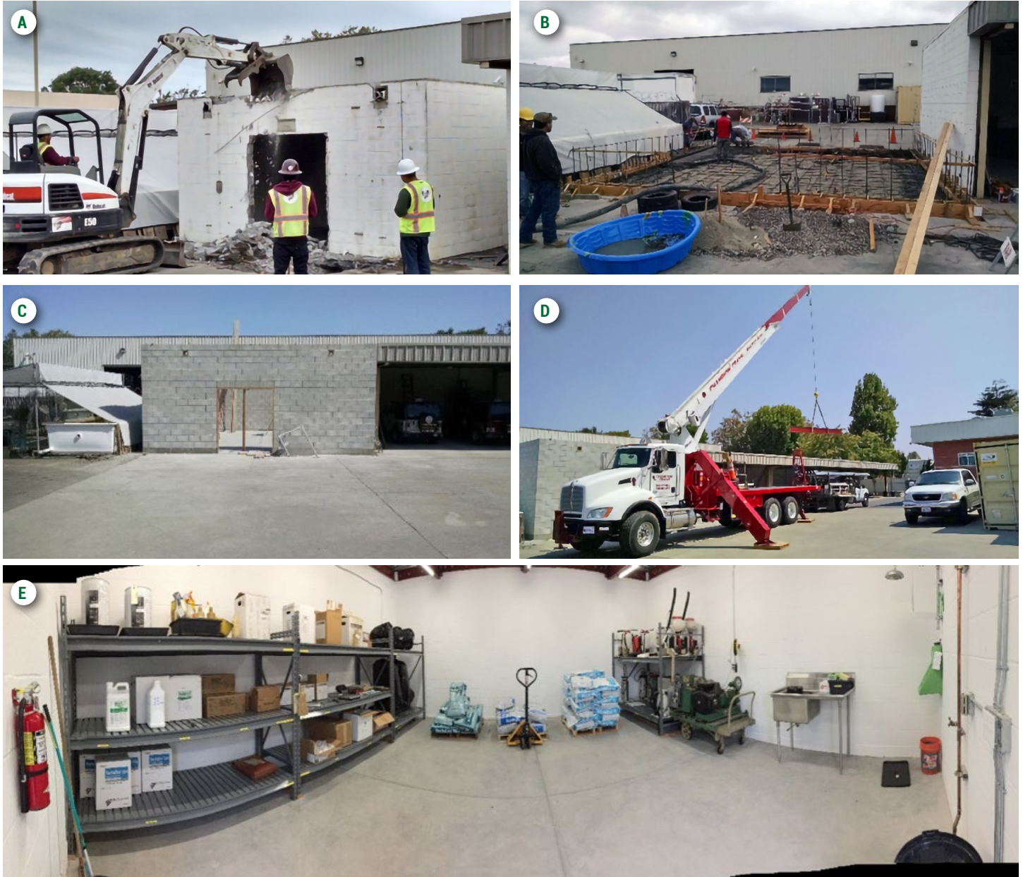
FIGURE 26: Pesticide storage shed remodel project
