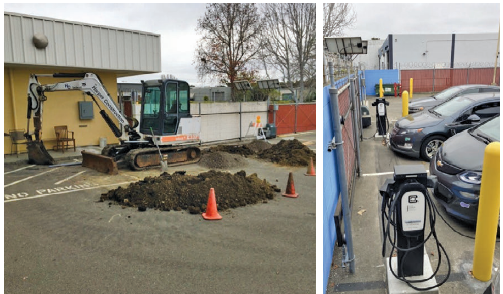
Figure 29. EV station intallations.
